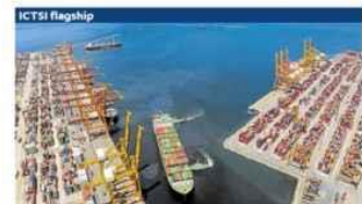
ICTSI flagship "GREEN PORT" Manila International Container Terminal, the Philippines' leading international trading gateway and flagship of International Container Terminal Services Inc., recently bagged the 2022 "Green Port Award" (GPAS) from the Asia-Pacific Economic Cooperation (Apec) Port Services Network. GPAS is an evaluation system for ports in the Apec region which recognizes "high caliber" and "sustainable" environmental actions and leadership. The award is valid for three years. —PHOTO FROM ICTSI
